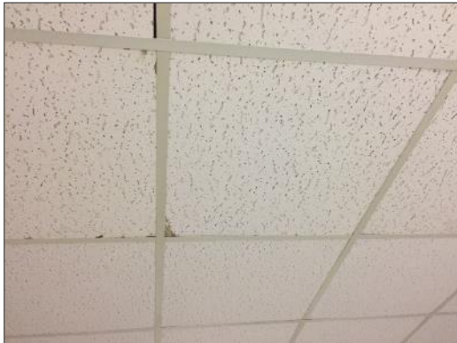
Asbestos-containing 24" x 24" lay-in ceiling tiles, large fissures and pinholes, Level 1 Corridor.
