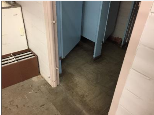
Photo 1 - Asbestos-containing 12" x 12" vinyl floor tiles, brown with thick brown lines, Basement Washroom adjacent to Housekeeping.
