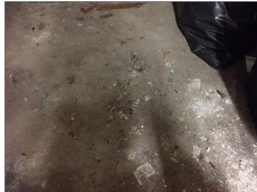
Photo 8 – Aircell debris on floor, Small Room in South Storage Room, M Wing Basement.
