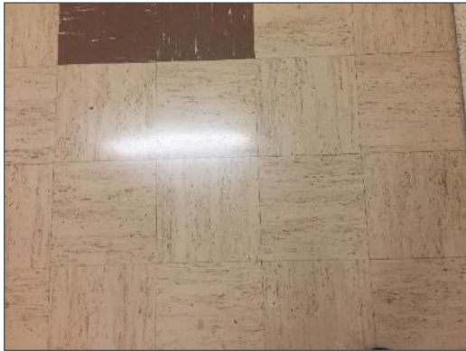
Photo 1 - Asbestos-containing 9" x 9" vinyl floor tiles, brown with thin brown lines, Level 1 E Wing North.
