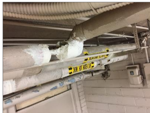
Photo 6 – Parging cement in fair condition, South Storage Room, M Wing Basement.
