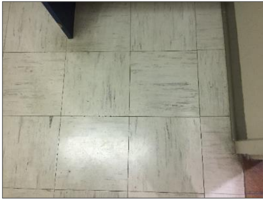
Non-asbestos 12" x 12" vinyl floor tiles and mastic, white with grey lines, Level 1 Women's Washroom.
