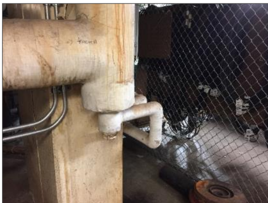
Asbestos-containing parging cement on pipe fittings, Basement Mechanical Room.
