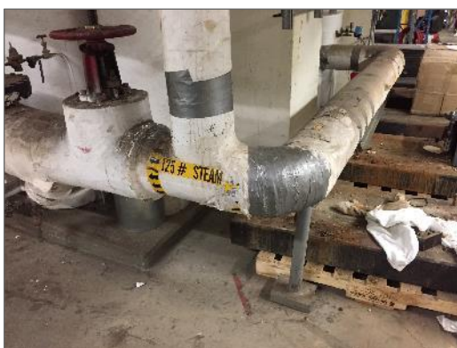
Photo 17 – Asbestos-containing parging cement in fair condition covered with duct tape at pipe fittings, 90 Wing E/F Basement Mechanical Room tunnel at Shop Area.
