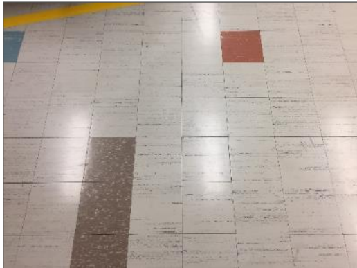
Photo 1 – Asbestos-containing 9" x 9" vinyl floor tiles, white with brown lines, Level 0 Corridor.
