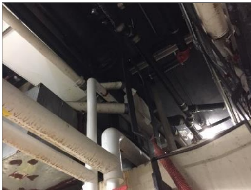
Photo 15 – Asbestos-containing parging cement in fair condition covered with duct tape at pipe fittings, 90 Wing E/F Basement Mechanical Room tunnel at Shop Area.
