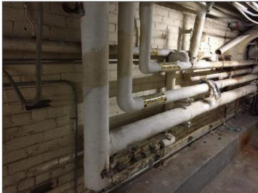
Asbestos-containing paring cement on pipe fittings, Basement Corridor.
