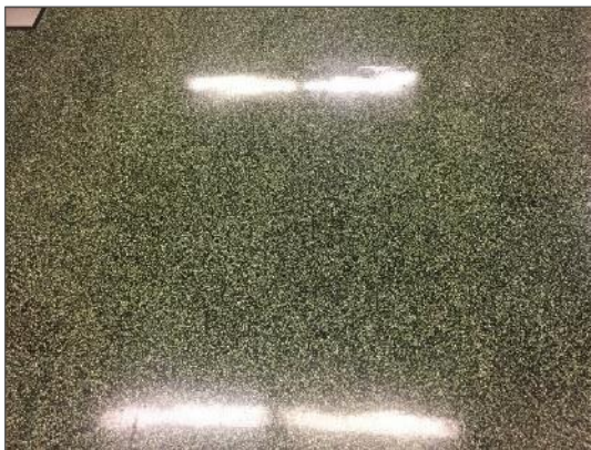
Photo 5 – Non-asbestos 9" x 9" vinyl floor tiles with asbestos-containing mastic, black and green flecks, E Wing Level 5 (North).
