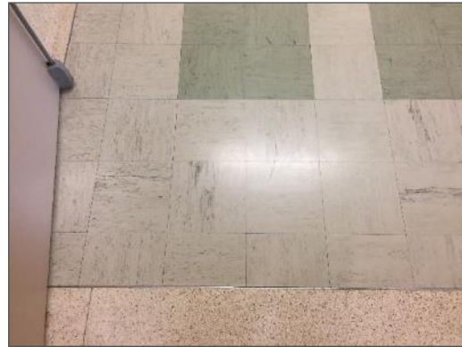
Photo 2 - Asbestos-containing 9" x 9" vinyl floor tiles, green with black flecks, Level 2 E Wing North.
