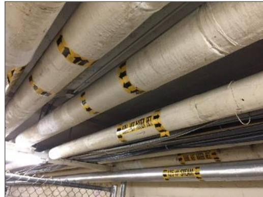
Asbestos-containing Aircell insulation on pipe straights, Basement Corridor.
