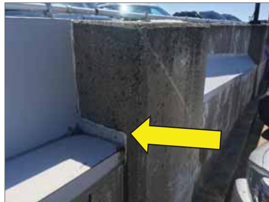
Asbestos-containing white caulking on panels, Level R
