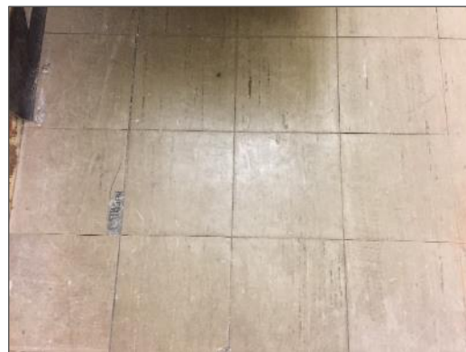
Photo 6 – Asbestos-containing 9" x 9" vinyl floor tiles, brown with white and brown lines, Level 0 Telephone Room.
