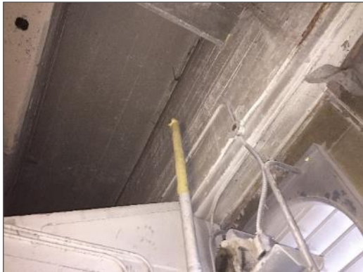
Photo 1 – Aircell in fair condition, Corridor at gate to R Wing, M Wing Basement.
