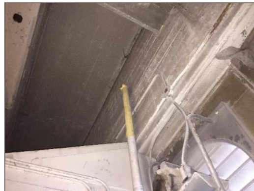
Asbestos-containing parging cement on pipe fitting, damaged condition, Upper Basement Level.
