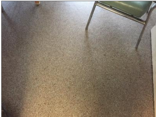
Non-asbestos vinyl sheet flooring, brown pebble pattern, Conference Room M1-32.
