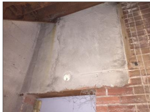
Non-asbestos rough plaster on metal lath, Middle Basement Level below stairs.
