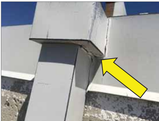
Asbestos-containing white caulking on eavestrough, Level R Elevator Lobby Roof
