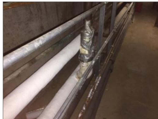
Photo 16 – Asbestos-containing parging cement in fair condition covered with duct tape at pipe fittings, 90 Wing E/F Basement Mechanical Room tunnel at Shop Area.
