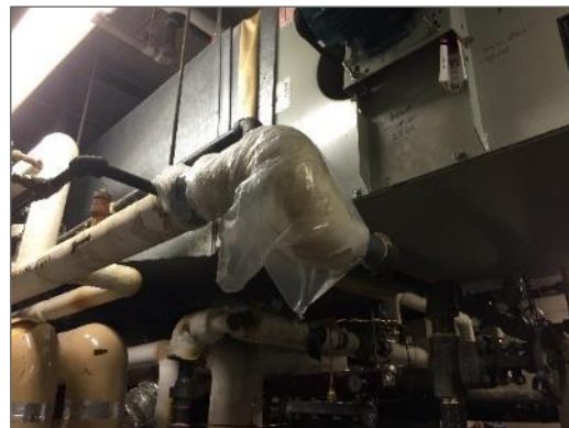
Photo 10– Asbestos-containing parging cement in fair condition covered with plastic wrap at pipe fittings, Level 0 G Wing Mechanical Room.
