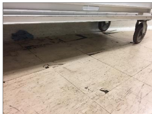
Photo 12– Asbestos-containing 12” x 12” vinyl floor tiles in poor condition, Level 0 Room 12, G Wing.
