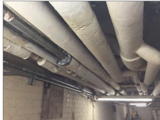
Photo 2 – Aircell in fair condition, West Corridor, M Wing Basement.
