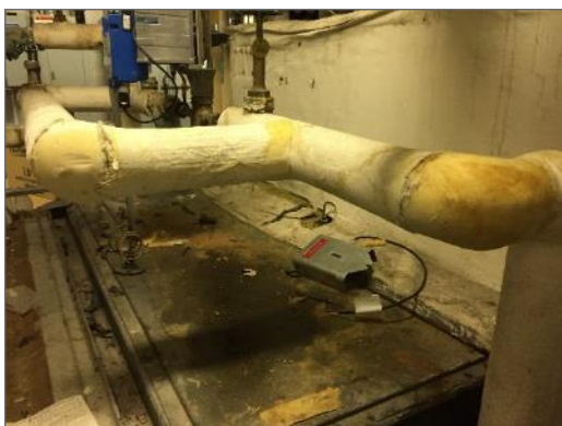
Photo 11 – Asbestos-containing parging cement in fair condition on pipe fittings, Level 0 G Wing Mechanical Room.
