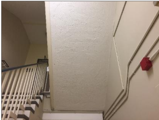
Asbestos-containing rough plaster on ceiling, Level 0 East Stairwell.
