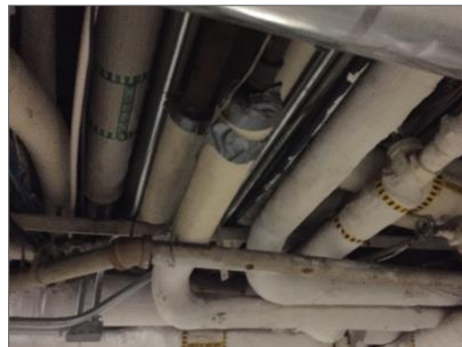
Photo 4 – Aircell in fair condition, Corridor near North Stairwell, M Wing Basement.
