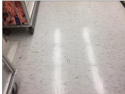
Photo 2 – Non-asbestos 12" x 12" vinyl floor tiles, white with black flecks, Level 0 Corridor.
