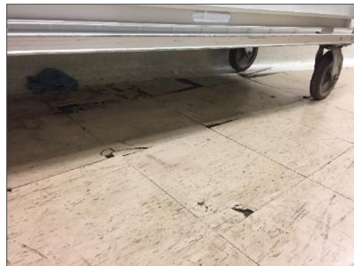
Photo 4 – Damaged asbestos-containing 12" x 12" vinyl floor tiles, brown with dark brown flecks, Room 12, Level 0.
