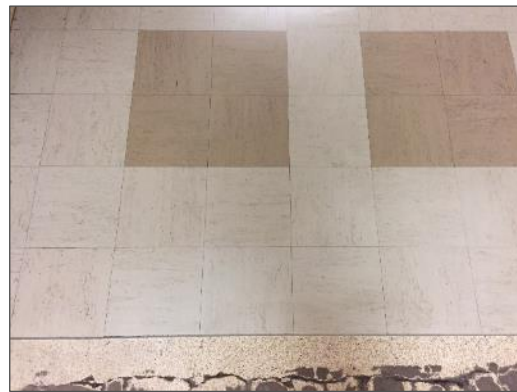
Photo 4 - Asbestos-containing 9" x 9" vinyl floor tiles, brown flecks, Level 2 E Wing Corridor North.
