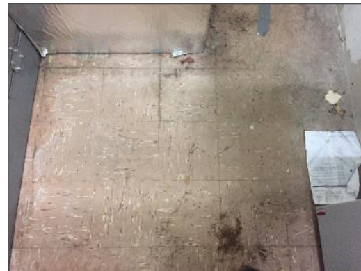
Photo 4 - Asbestos-containing 9" x 9" vinyl floor tiles, brown flecks, Level 0 North Entrance.
