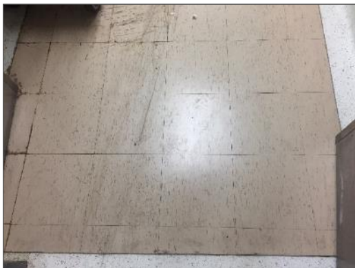
Photo 3 – Asbestos-containing 12" x 12" vinyl floor tiles, brown with dark brown flecks, Room 12, Level 0.
