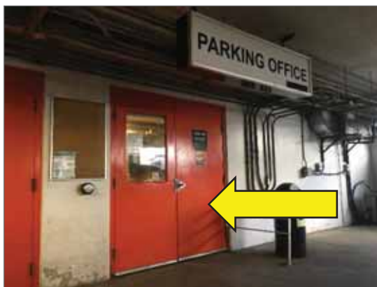
Lead-containing orange paint on metal door, Parking Office
