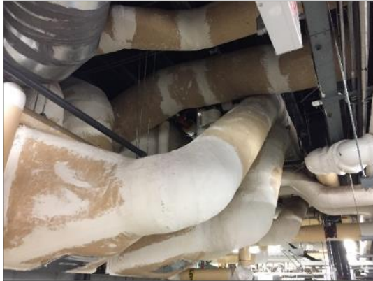
Asbestos-containing parging cement on ducts, Penthouse.
