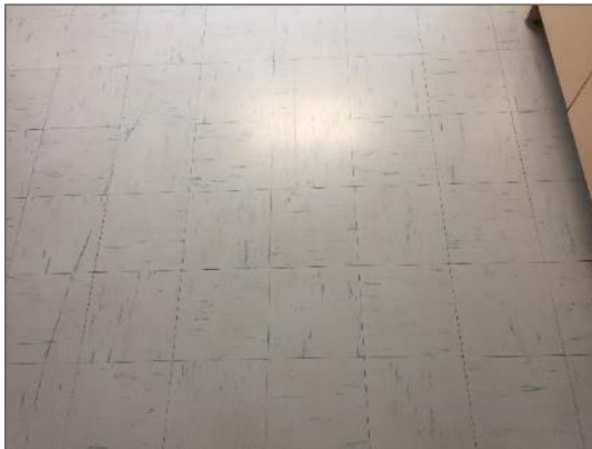
Photo 3 - Asbestos-containing 9" x 9" vinyl floor tiles, white with blue lines, Level 2 E Wing North Lounge.
