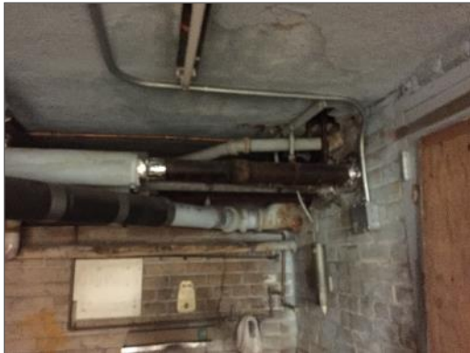
Photo 7 – Taped ends of Aircell in fair condition, South Storage Room, M Wing Basement.
