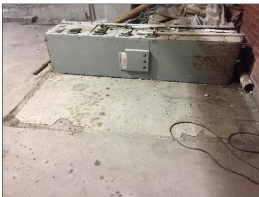
Asbestos-containing 12" x 12" vinyl floor tiles, beige fleck pattern, Lowest Basement Level.
