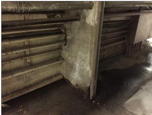
Non-asbestos rough plaster partition wall, Basement Tunnel to Boiler House.
