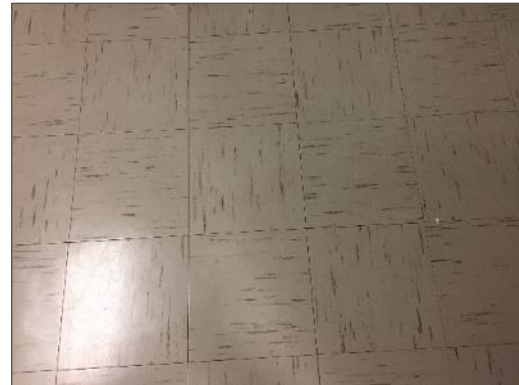
Photo 2 - Asbestos-containing 12" x 12" vinyl floor tiles, white with brown lines, Level 0 Central Media Lab Office.
