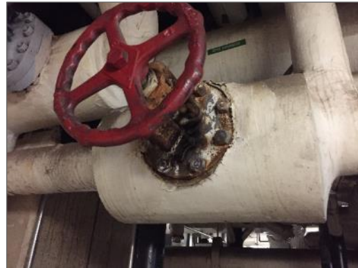
Photo 14 – Asbestos-containing parging cement in fair condition at pipe fitting, 90 Wing E/F Basement Mechanical Room near column R22.
