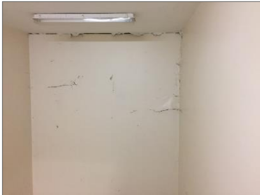
Photo 13 – Damaged asbestos-containing plaster on ceiling, Level 4 G Wing East Stairwell.
