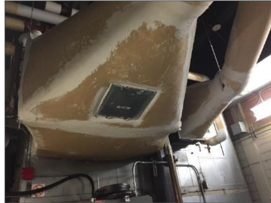
Asbestos-containing parging cement on ducts, Penthouse.
